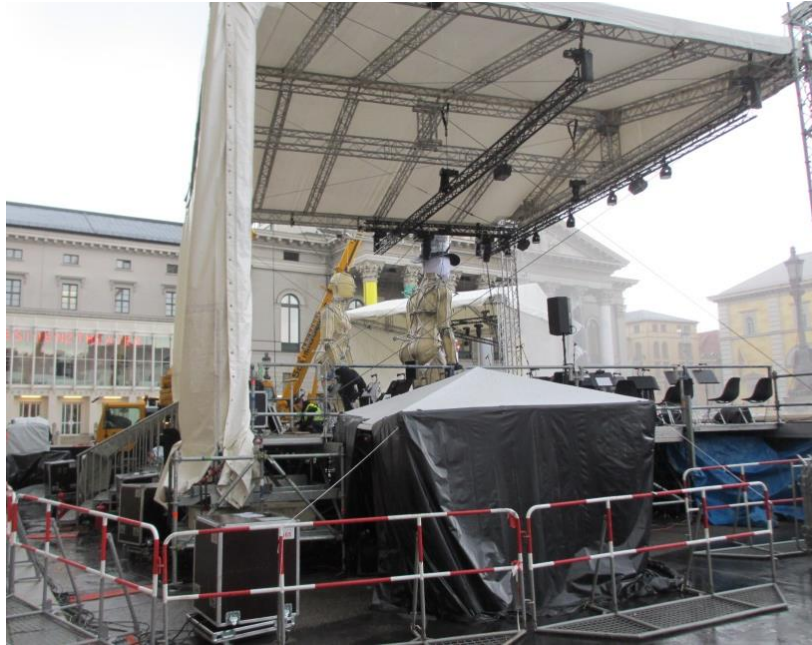
A construction site across from the State Opera featured two giant boxing robots.
